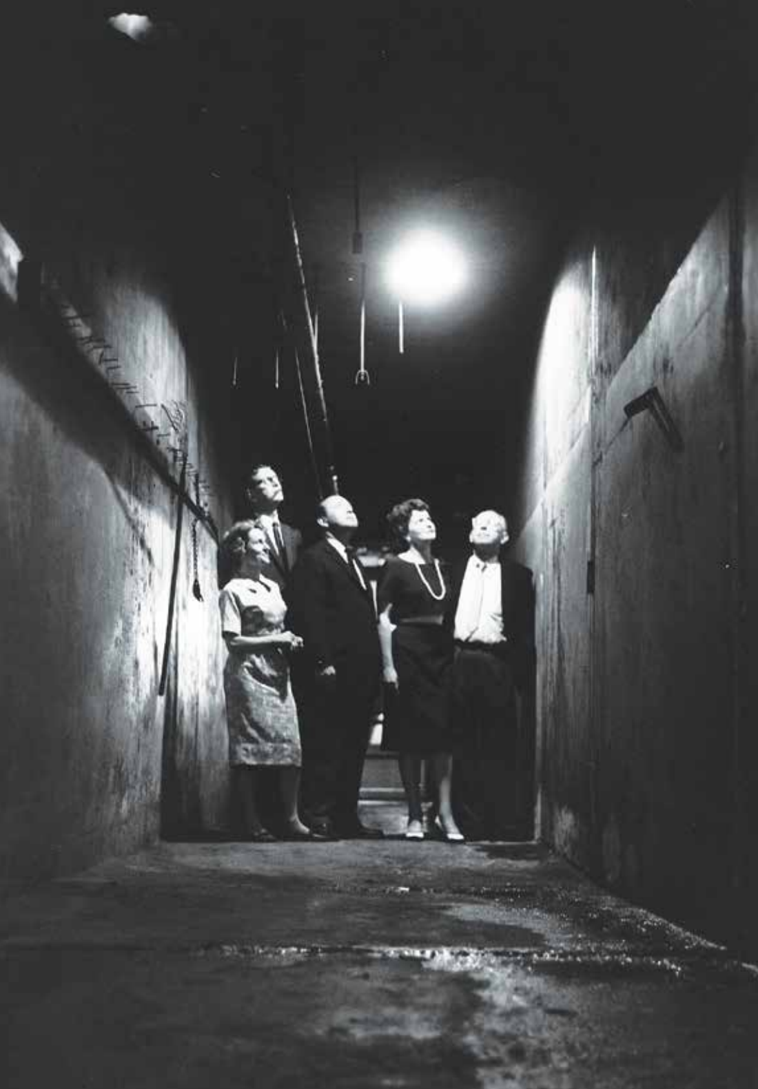
BBAC Archival Photo: In the BBAC Tunnel
